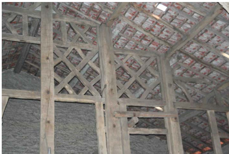
Charpente de la grange de Béning. Ph. Jean-Marie Blaising.
